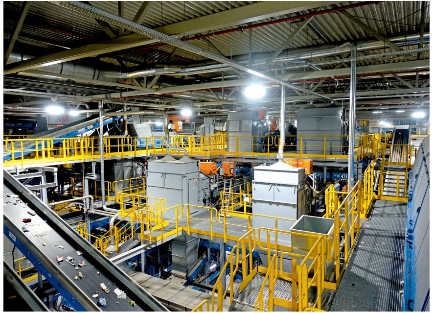
View into the IVAR plant: since 2019, 22 autosort machines are sorting plastics and paper here.
